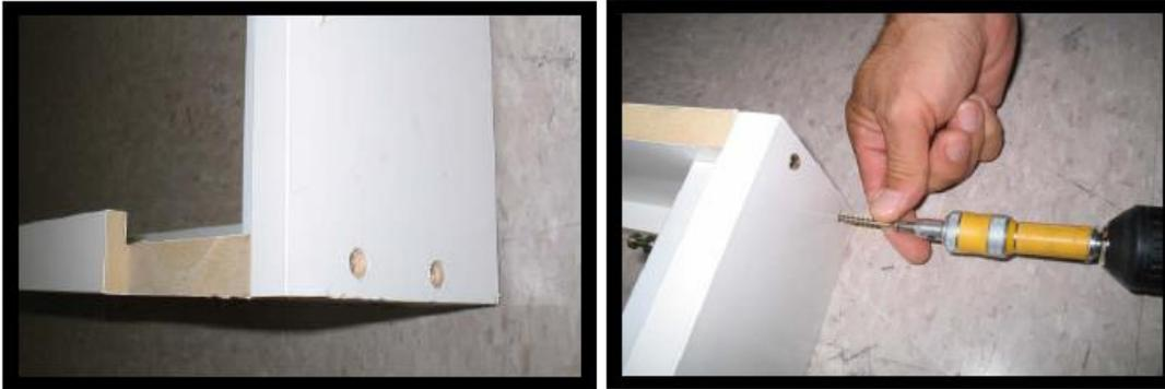
4. Place and position the assembled frame **EVENLY** around the window opening. Screw **ONLY** the upper left and right corners of the side box frame to the wall or window recess
